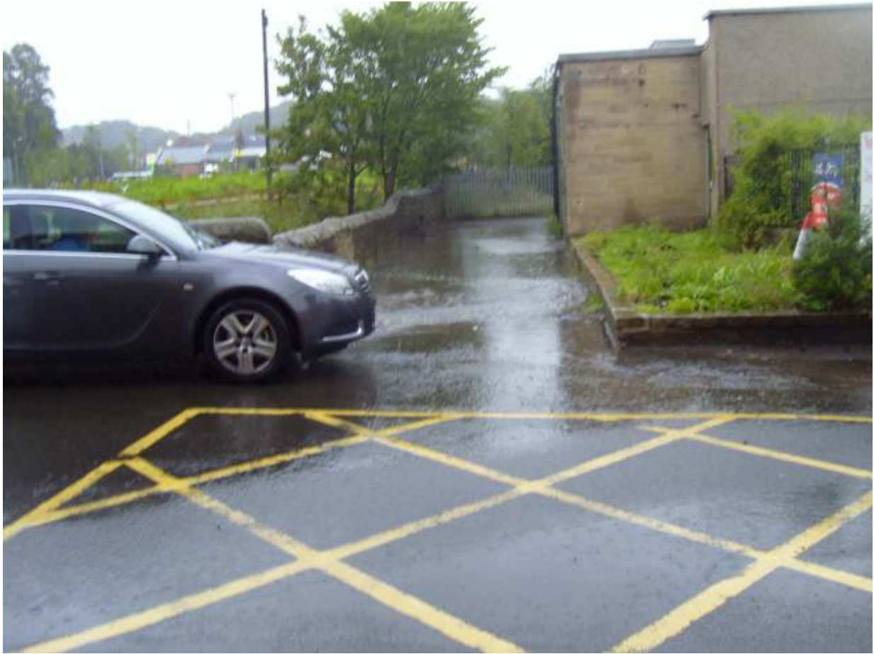
An electricity supply company engineer arrives to monitor the flooding of the substation
