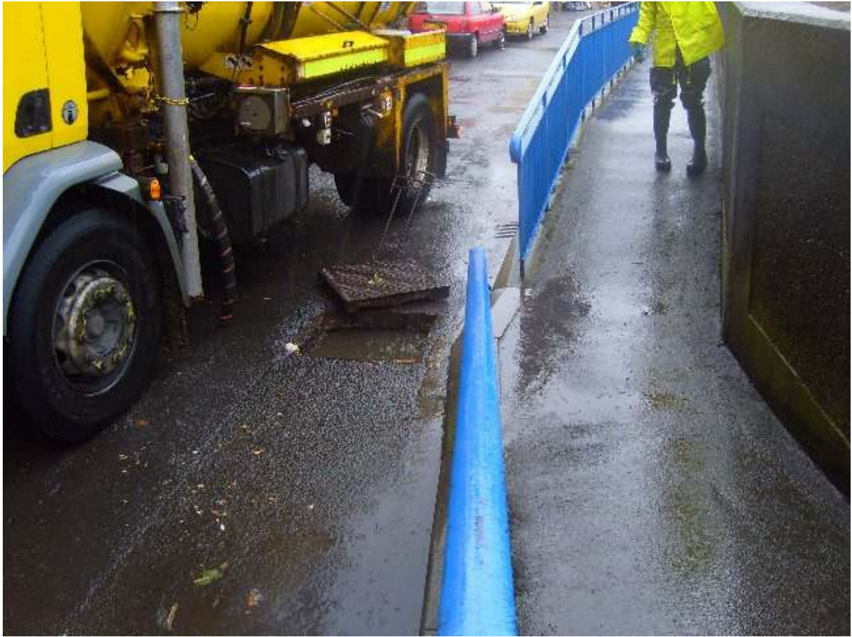
Northumbrian Water manhole full to overflowing Bennetts Walk 17 th July 2009
